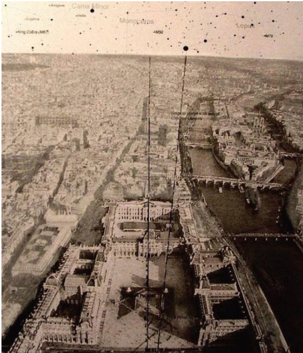
f 13. Aerial view of the Historical Axis of Paris looking west from the Louvre towards La Défense on the distant horizon. Note the deviation of the axis.
